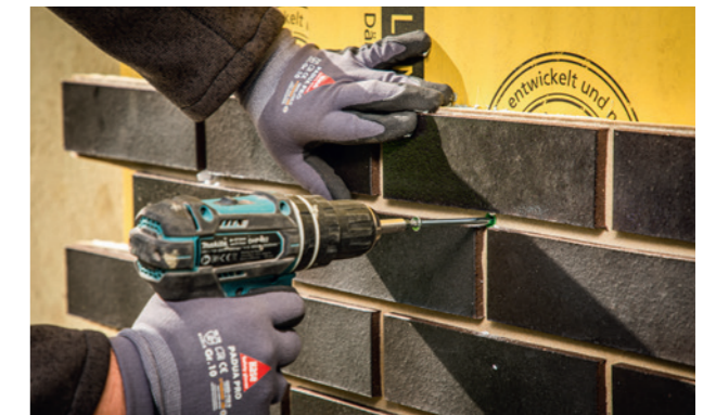
Step 7: Fastening the elements
