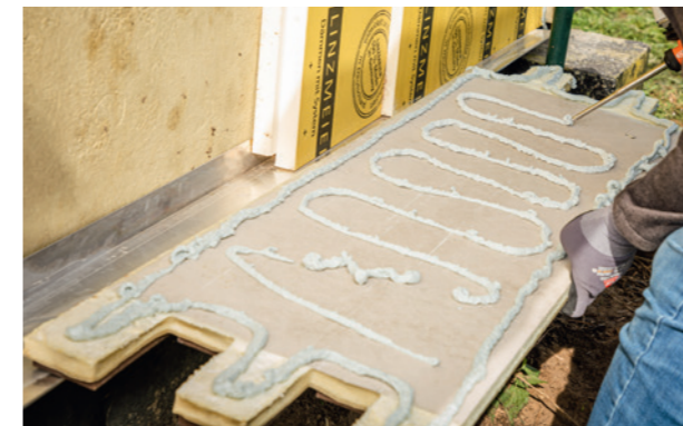
Step 4: Applying foam to the elements
