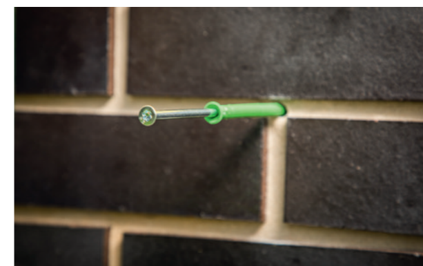
Step 6: Drilling for fixings; setting suitable plugs and screws
