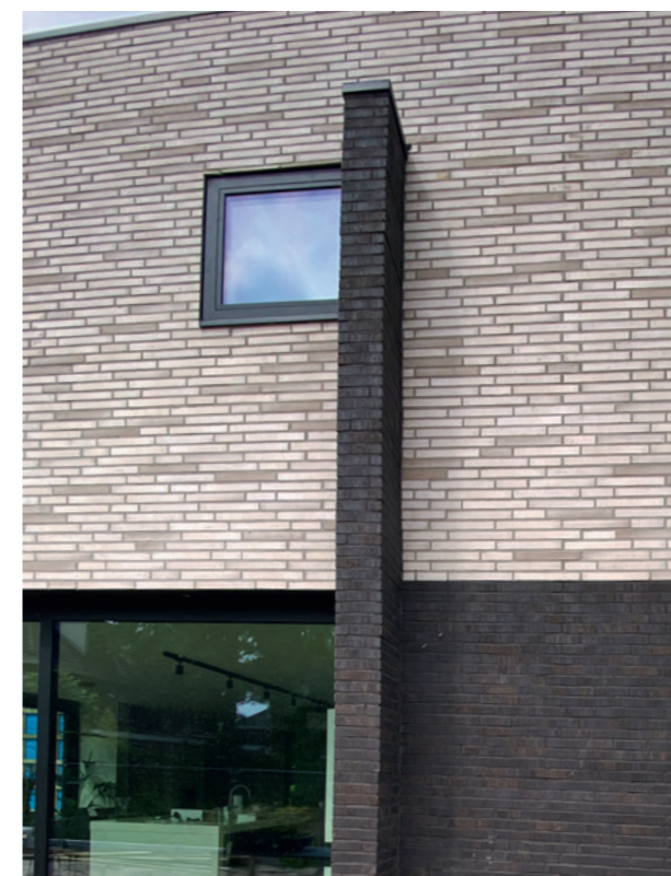
Wild bond with grey bricks on an office/residential building with a half column
