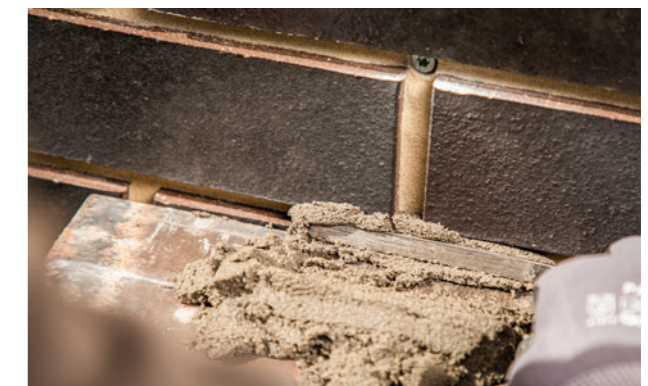
Step 8: Grouting the brick facade
