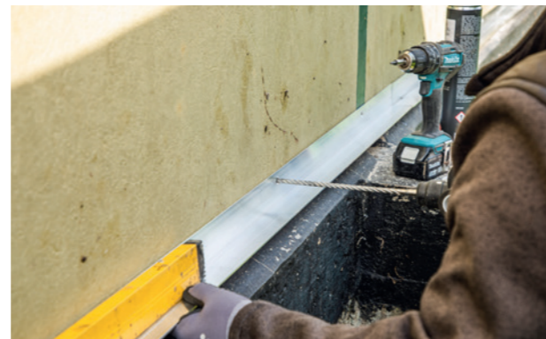
Step 1: Setting the starter rail (optional)
