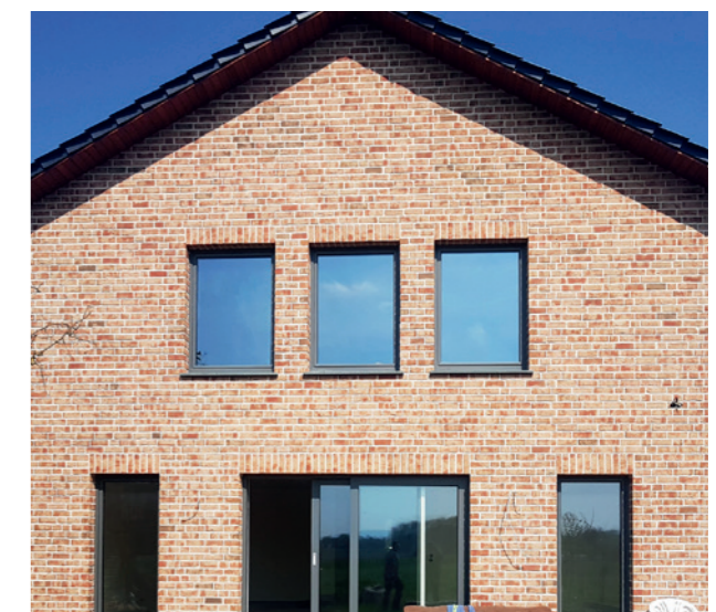
U-shaped elements are also a speedy and effective cladding solution when windows are close together.
