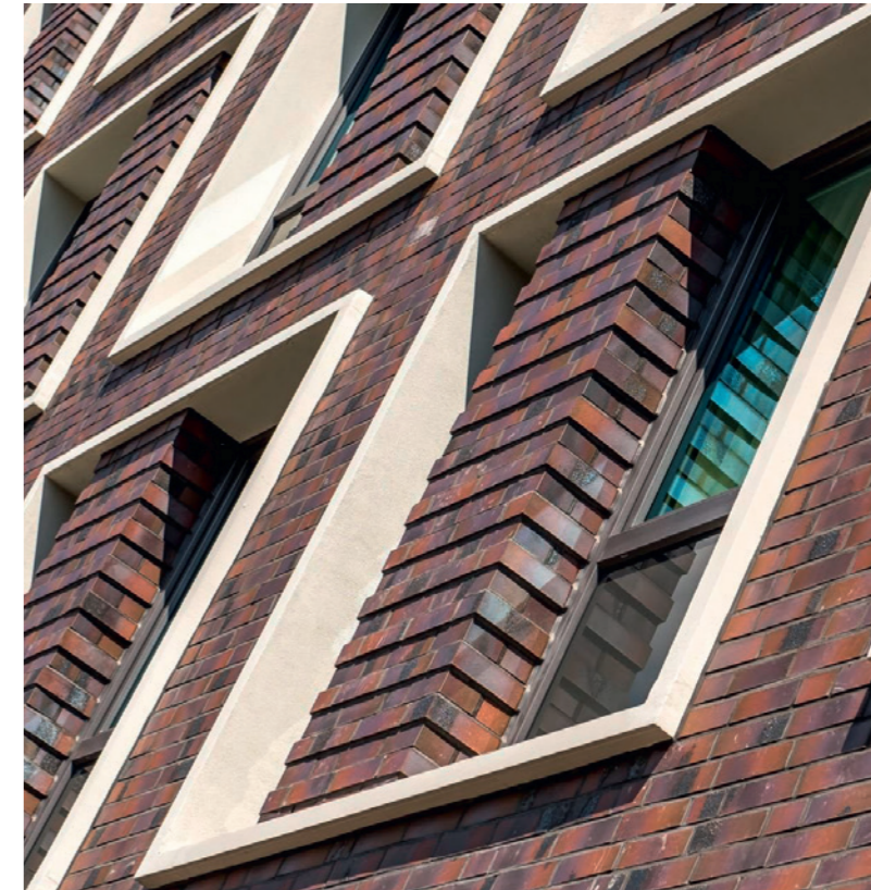
Protruding, plastered window reveals contrast beautifully with the brick facade.
