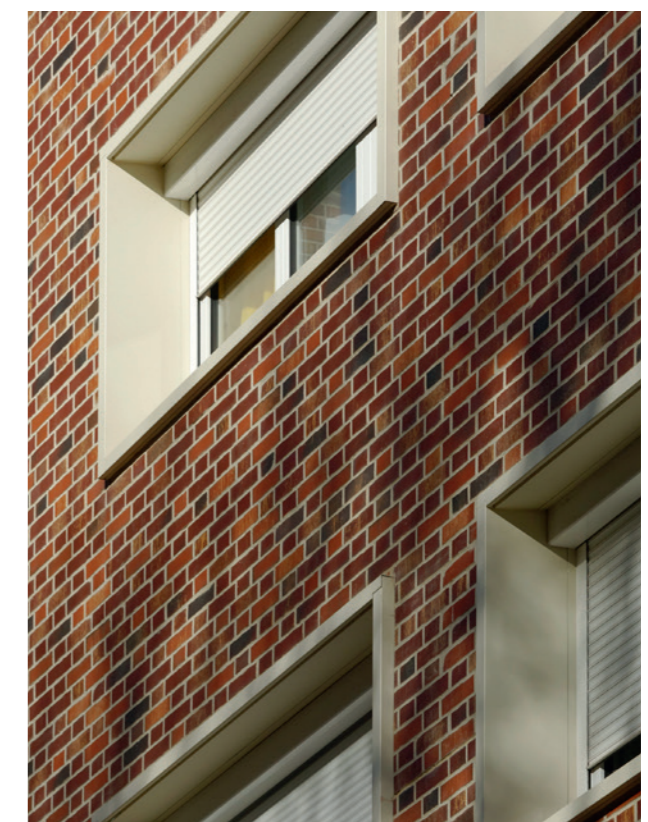
Dark red bricks in Flemish bond
