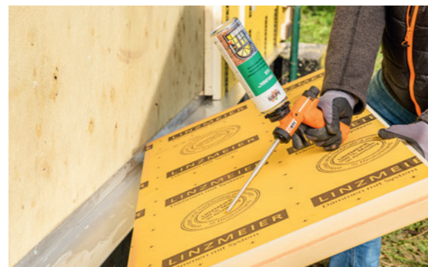
Step 2: Attaching the insulation
